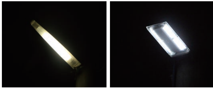
a. Fluorescent Lights (Inverter-type and Starter-type)
